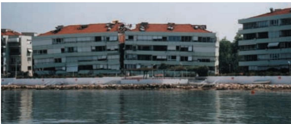
Apartment block split in two by the 1999 earthquake in Izmit, Turkey
