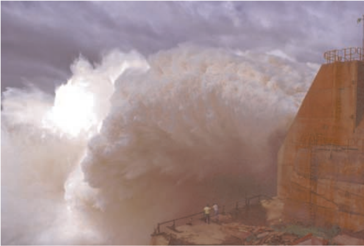
One of the world's largest dams — the Itaipu hydroelectric plant in Brazil. The future of such projects is called in question by a new report
